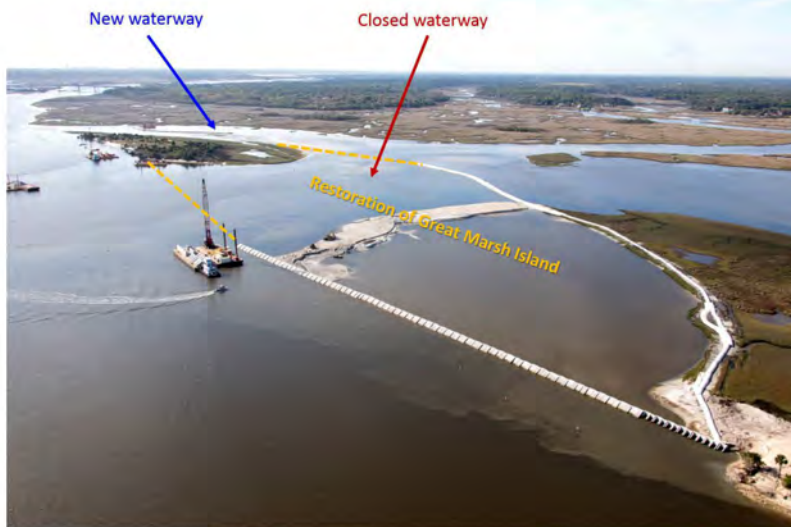
Mile Point Construction (Photo by Mark Bias)
