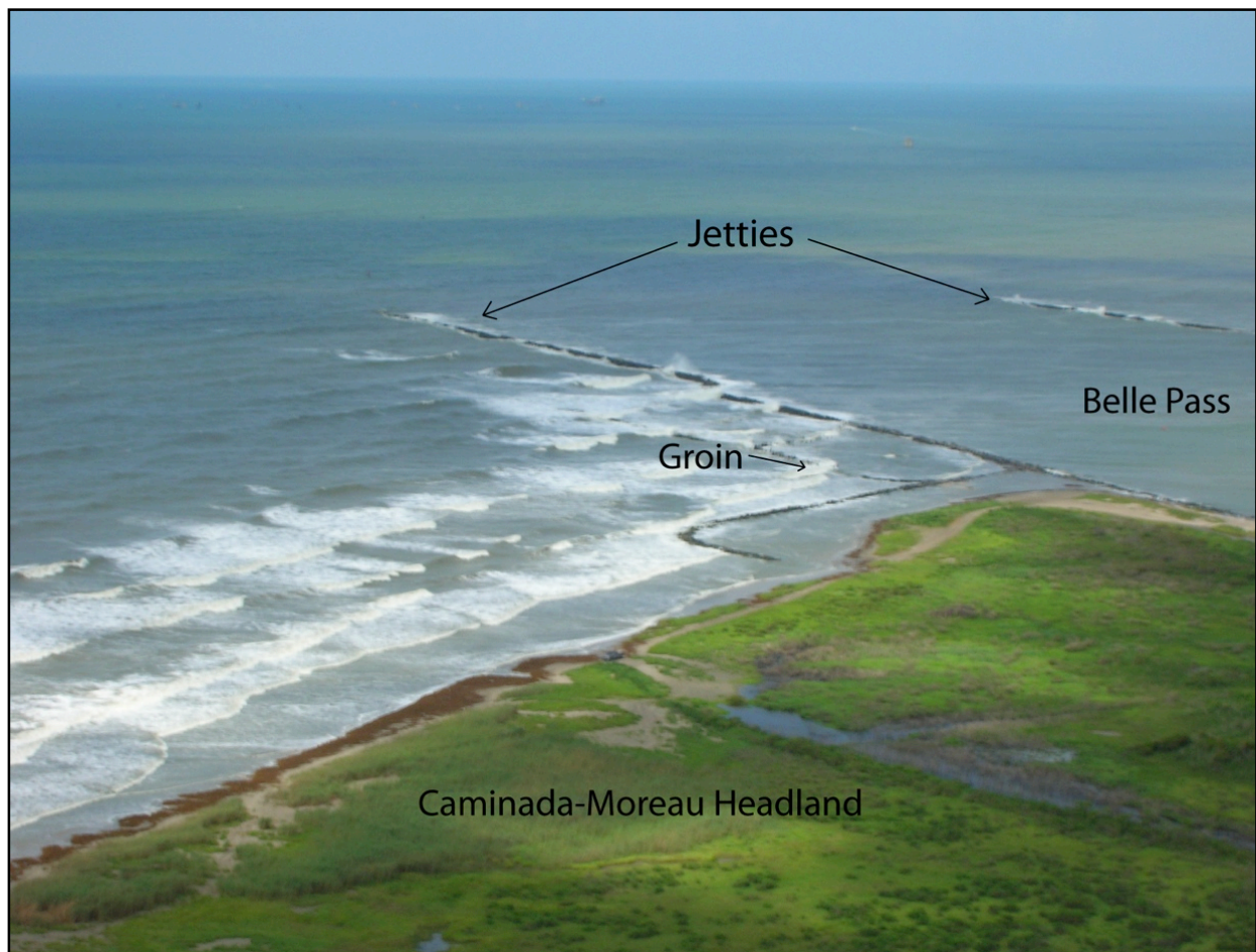
Figure 5: Oblique aerial view of the Belle Pass jetties and groin taken after Hurricane Cindy (Cat. 1) landfall on the Caminada-Moreau Headland on July 11, 2005. (Image credit D. Weathers).
