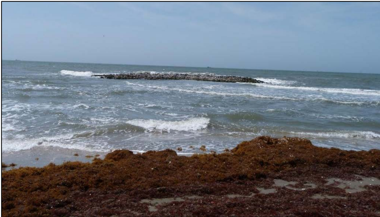
Figure 6: Rocks initially placed on the bayside of East Timbalier currently function as a breakwater off the Gulf-side shoreline. (Curolle et al., 2012.)
