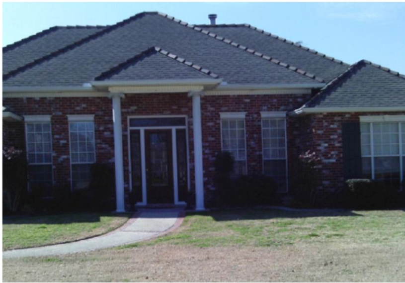
~ 6 feet below BFE
