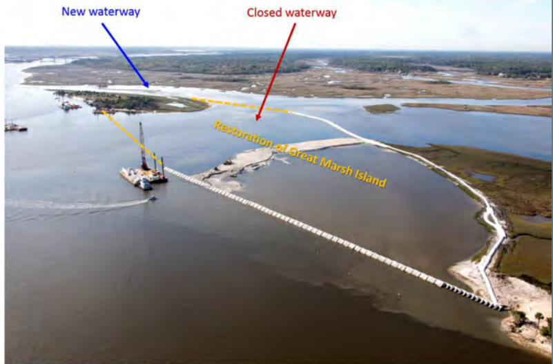
Mile Point Construction (Photo by Mark Bias)
