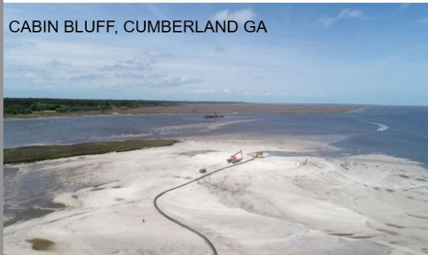
top of berm was designed to be ~+10ft MLLW with a 1 on 15 slope
