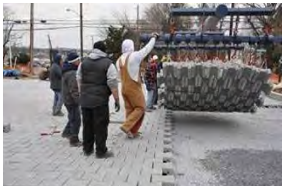
Left: Permeable Articulating Concrete Block Pavers
