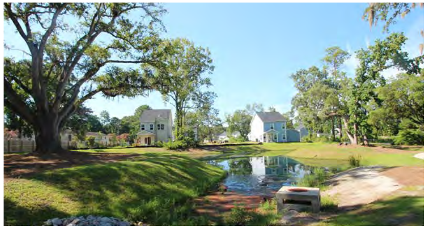
Low Homes in the Lower Basin New slab-on-grade developments near the mouth of the creek.
