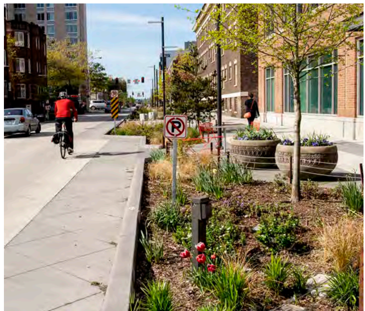
Bioretention Planter Alongside Bell Street, Seattle, WA
