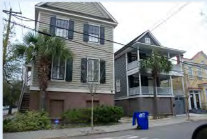
Solid foundation at front
