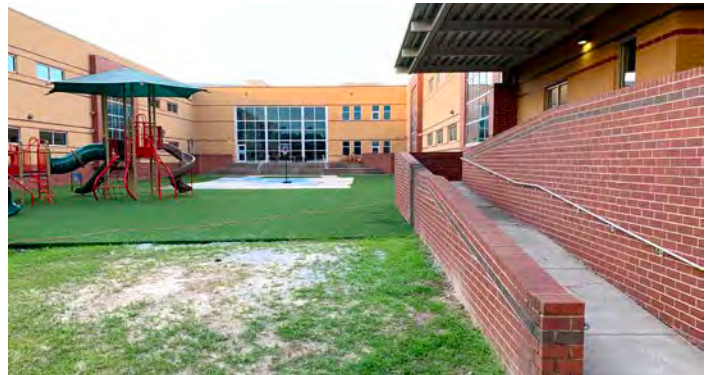
Sanders Clyde Elementary School Potential for water management and educational interventions in courtyard and open spaces
