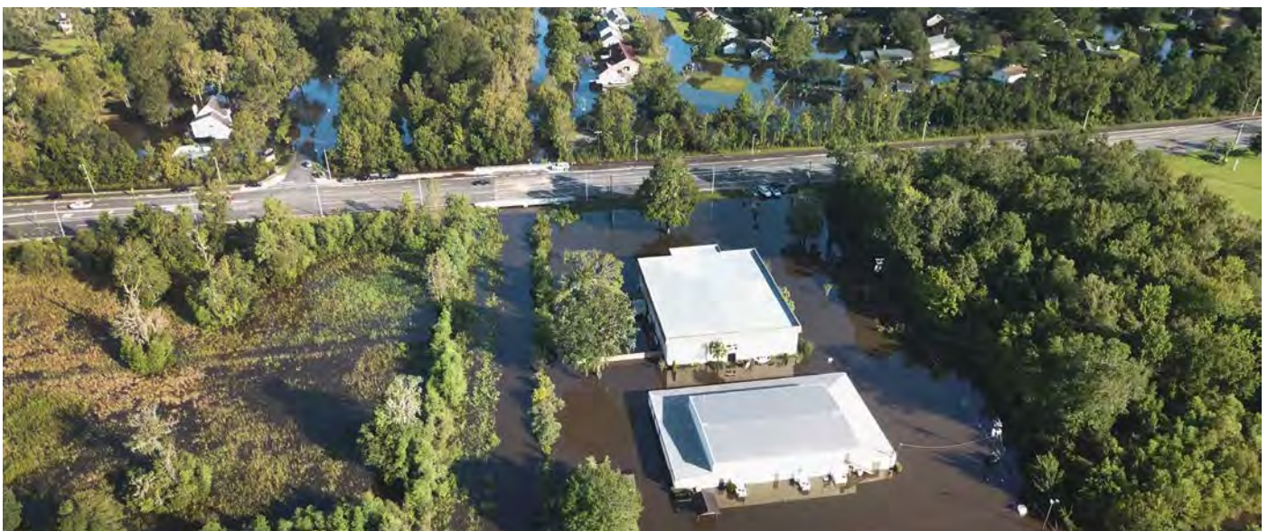
Flooding at Bees Ferry Road and Church Creek Intersection Crosstowne Church (pictured) has flooded multiple times in the last 5 years.
