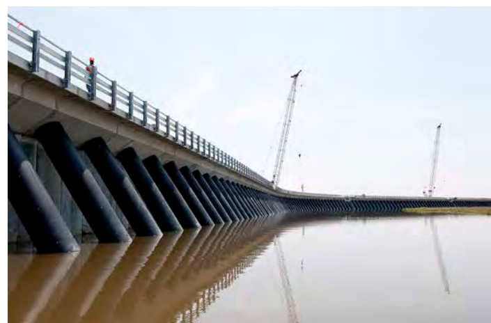
New Orleans Inner Harbor Navigation Channel Surge Barrier
