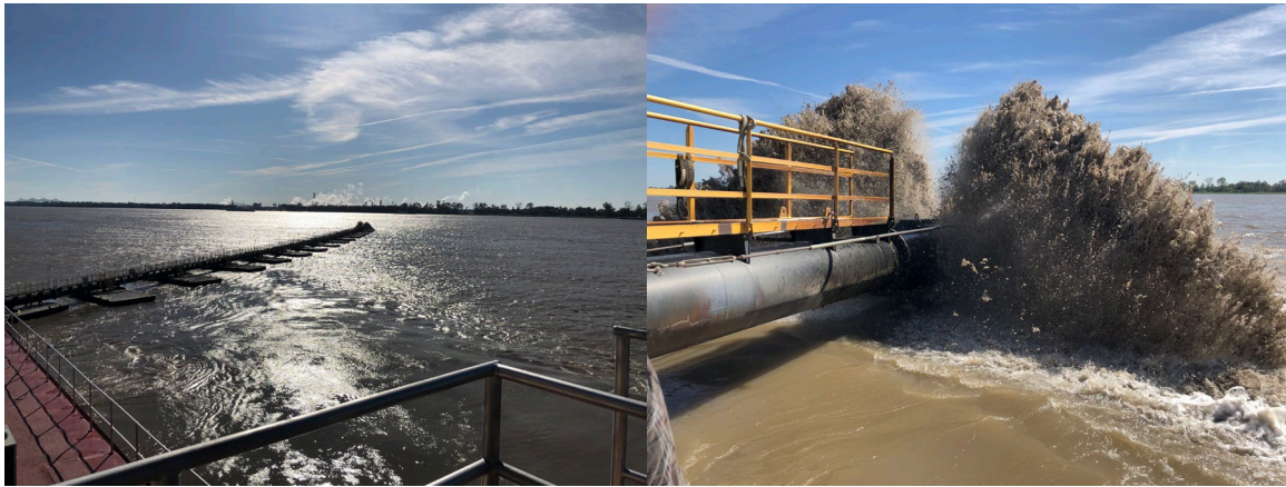
Figure 13. Discharge pipeline (left) and end of discharge pipeline with baffle plate diffusing material (right). Images taken aboard the USACE Dredge Jadwin operating at Smoke Bend Crossing.
