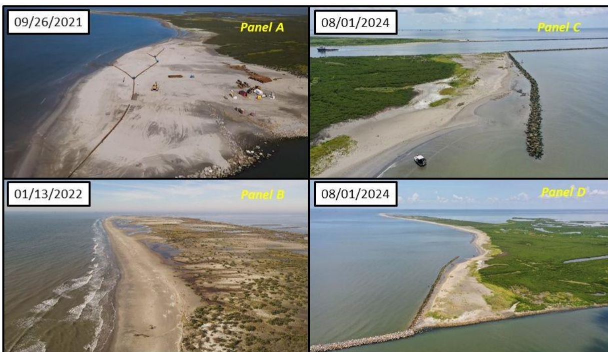
Figure 16. Drone imagery showing feeder beach construction (top left), feeder beach post-completion detailing longshore sediment transport (bottom left), and evidence of shoreline retreat and revetment exposure immediately west of Belle Pass jetties (top right and bottom right). Imagery provided by CPRA.
